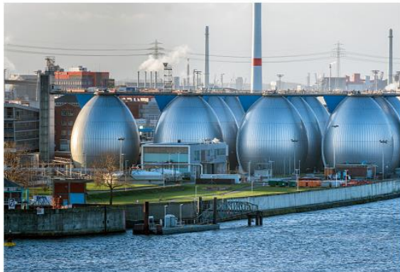
Desalination by distillation in Hamburg Germany
